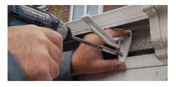
3 Ensure bracket is vertically aligned and secure with self-drilling screws through two remaining holes.
