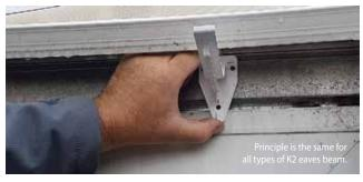
2 Insert a galvanised steel self-drilling screw through the bottom hole and drill to fix in place.
