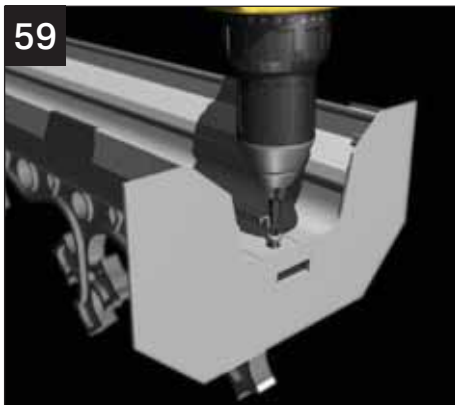
59 Screw the flashing trim to the ridge top cap through the screw port. Use a 4.2mm x 13mm self drilling screw (not supplied).
