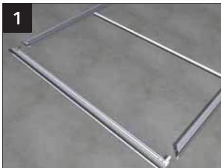
1 Layout the pieces of the lantern eaves beam.
